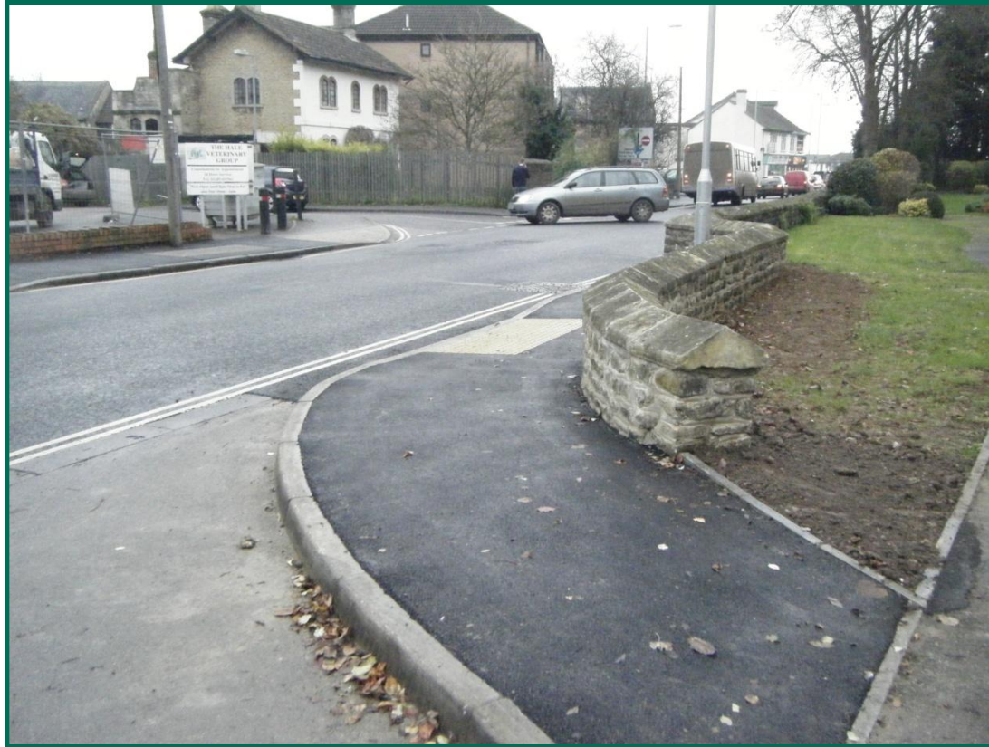
Langley Road - Footway Link & crossing point AFTER
